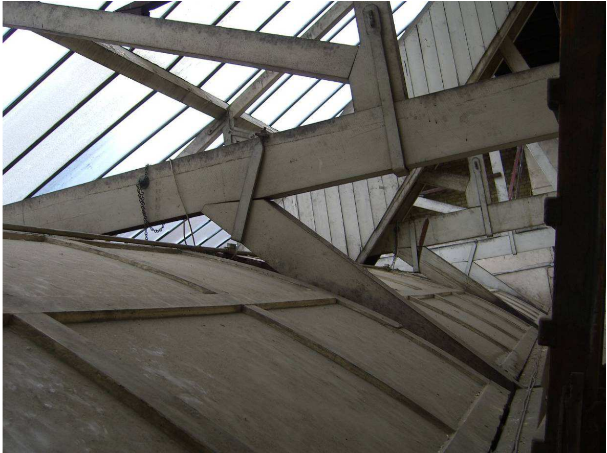
Photo 7. Roof void between roof light and glazed vault over ground floor
