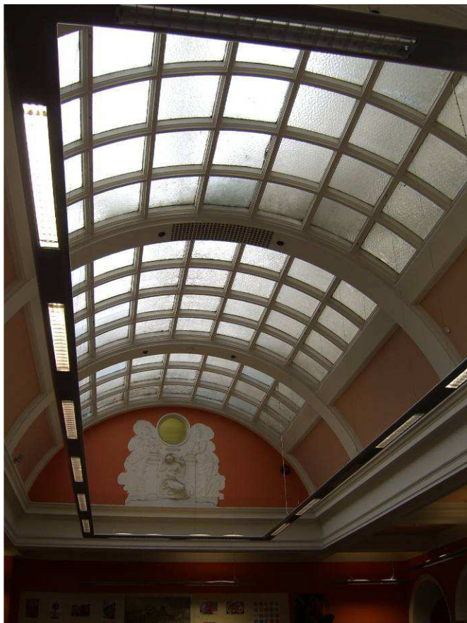
Photo 8. Glazed vault over main ground floor area of library
