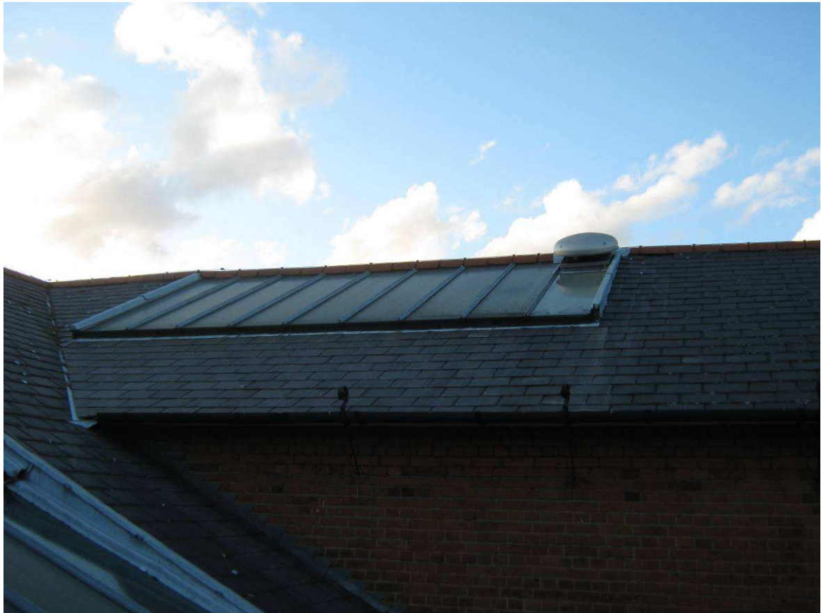
Photo 3. Roof light over reference library
