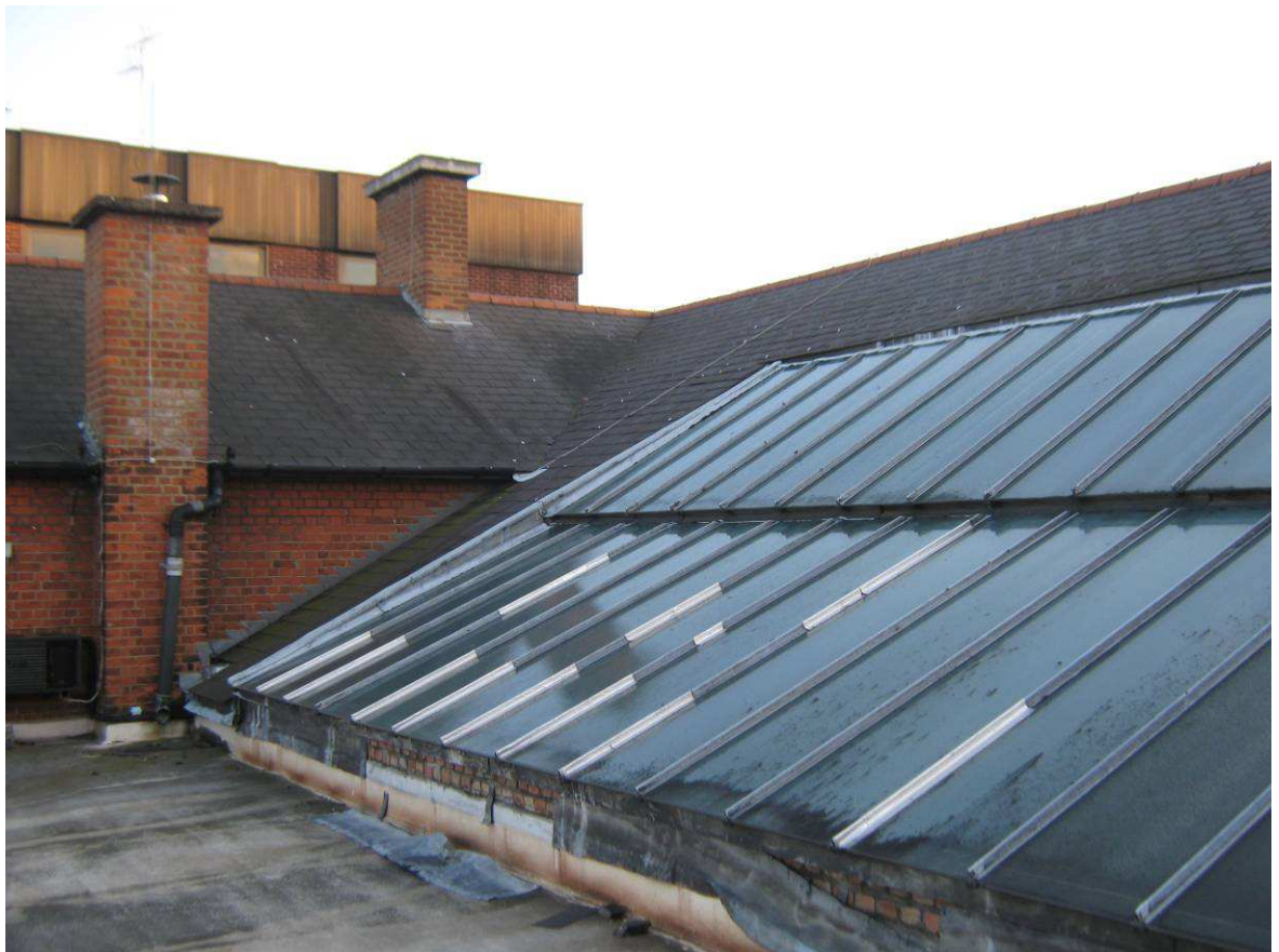
Photo 2. Roof light over glazed vault to ground floor
