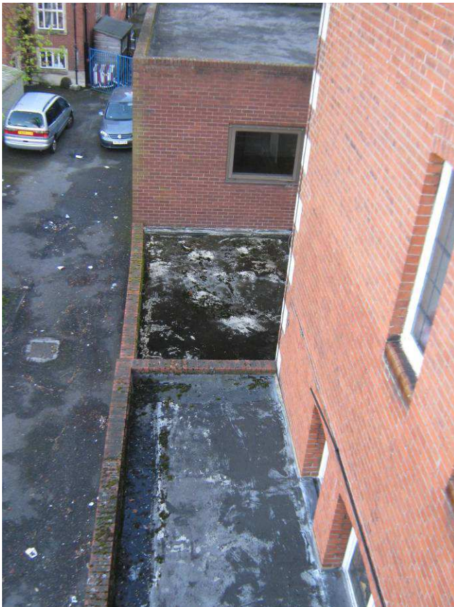
Photo 6. Flat roof over the staff entrance
